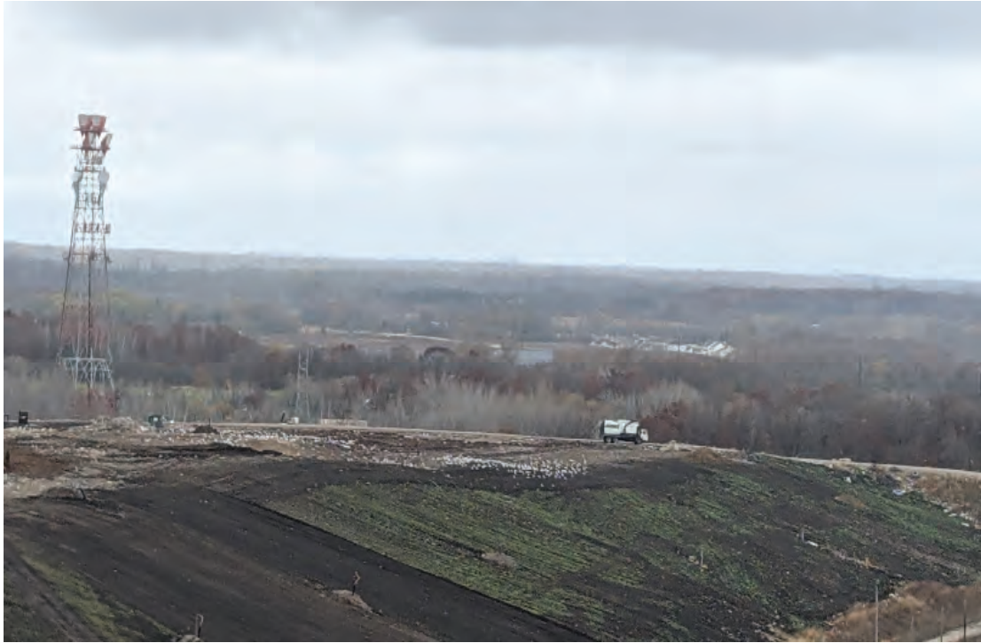
Top soil on Phase 1 slopes greening up with vegetation
