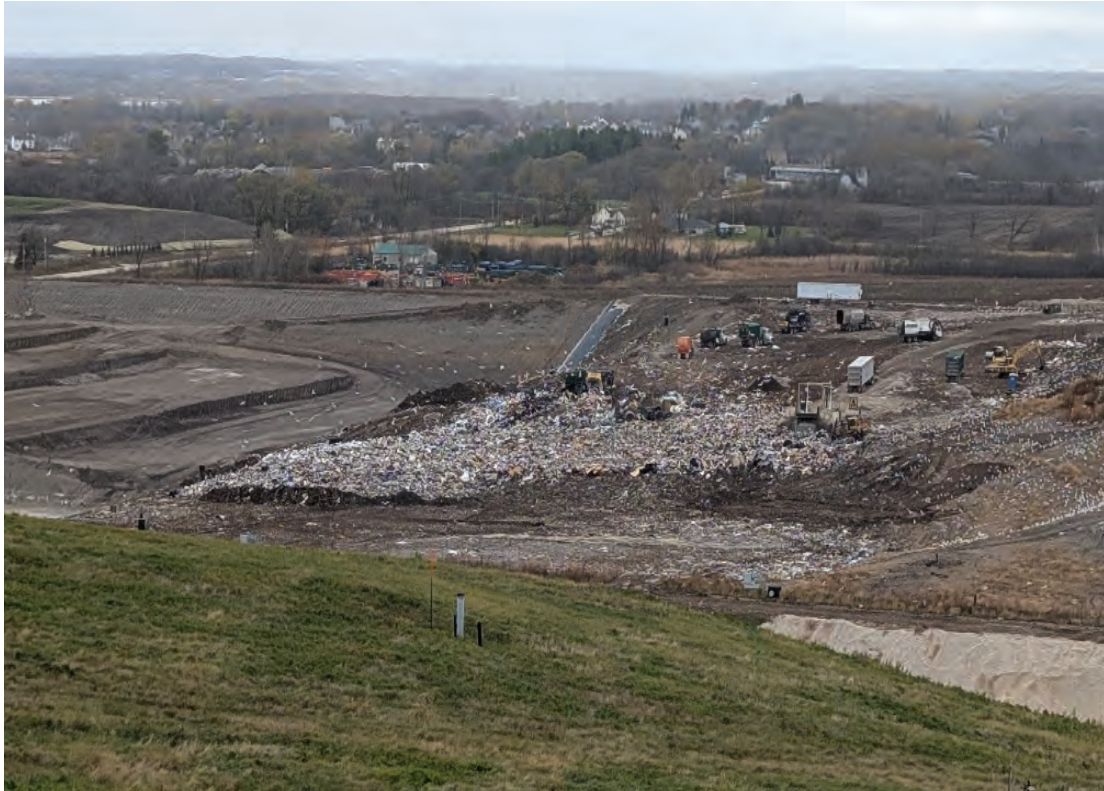
Working face at South end of Phase 3, shaping waste for cell slopes and cover being placed as elevations/slopes are reached
