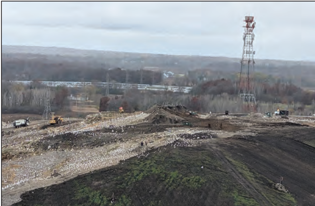
Cover soil stockpile on top of Phase 1/2
